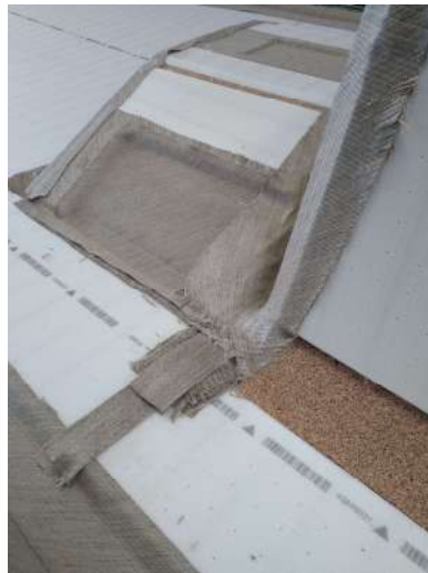
Draping of the deck
